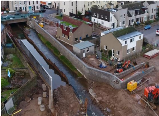
4A Flood Walls and Beach Bridge abutment
