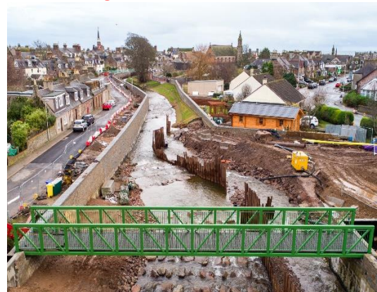
Green Bridge, flow control and Flood Walls
