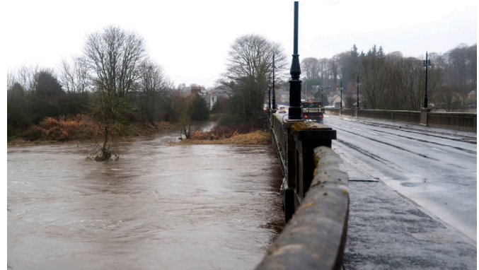
High water levels River Don - Flooding at Kintore, Port Elphinstone, Inverurie
