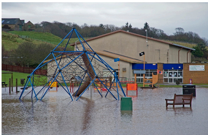
Flooding outside Stonehaven leisure centre
