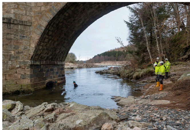
Potarch Bridge divers carrying out an underwater bridge inspection
