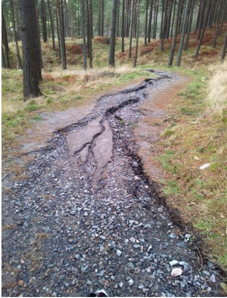
Scour on path at West Wood
