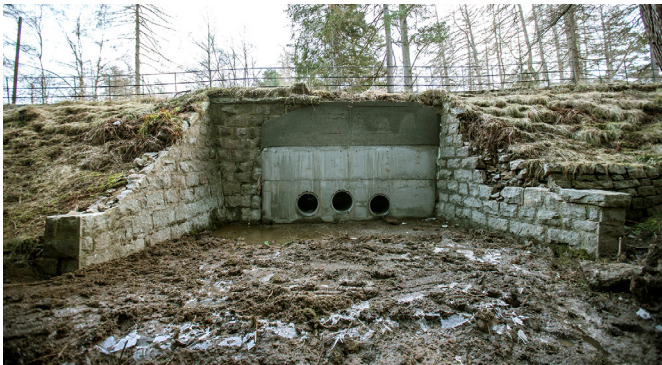
Repair works to Invercauld Bridge, reconnecting Braemar
