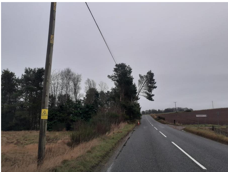
Tree being held up by an HV cable B993 Craigeam in November 2021
