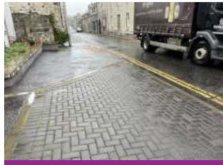
“Narrow roads and pavements are dangerous for pedestrians.”
