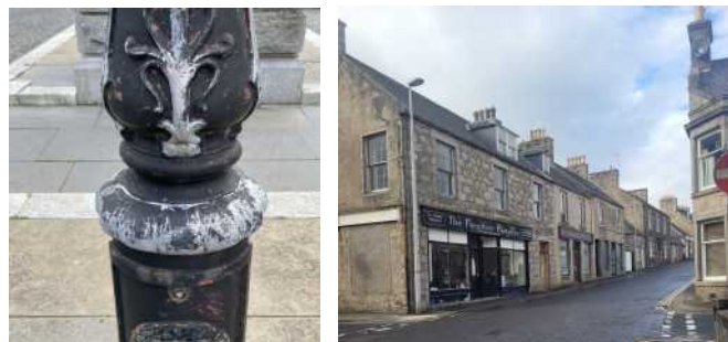
Images (Clockwise from Top Left): Some maintenance required; Standard LED lighting, Duke Street; Mixture of traditional lighting styles in the Square.
