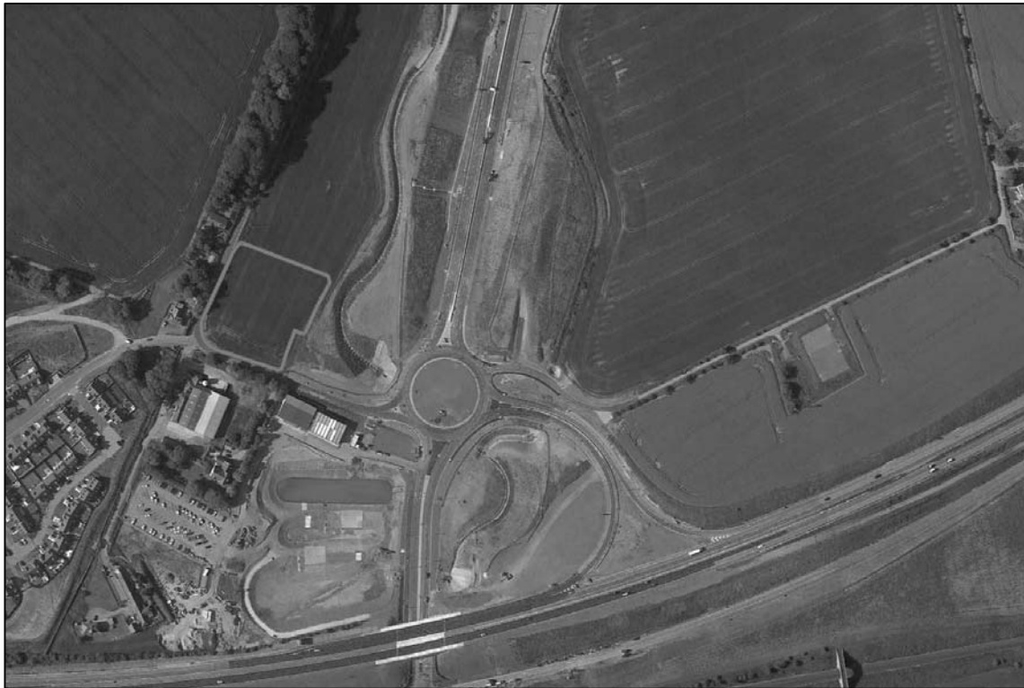
Figure 6 – Aerial Photograph of Site KN118
