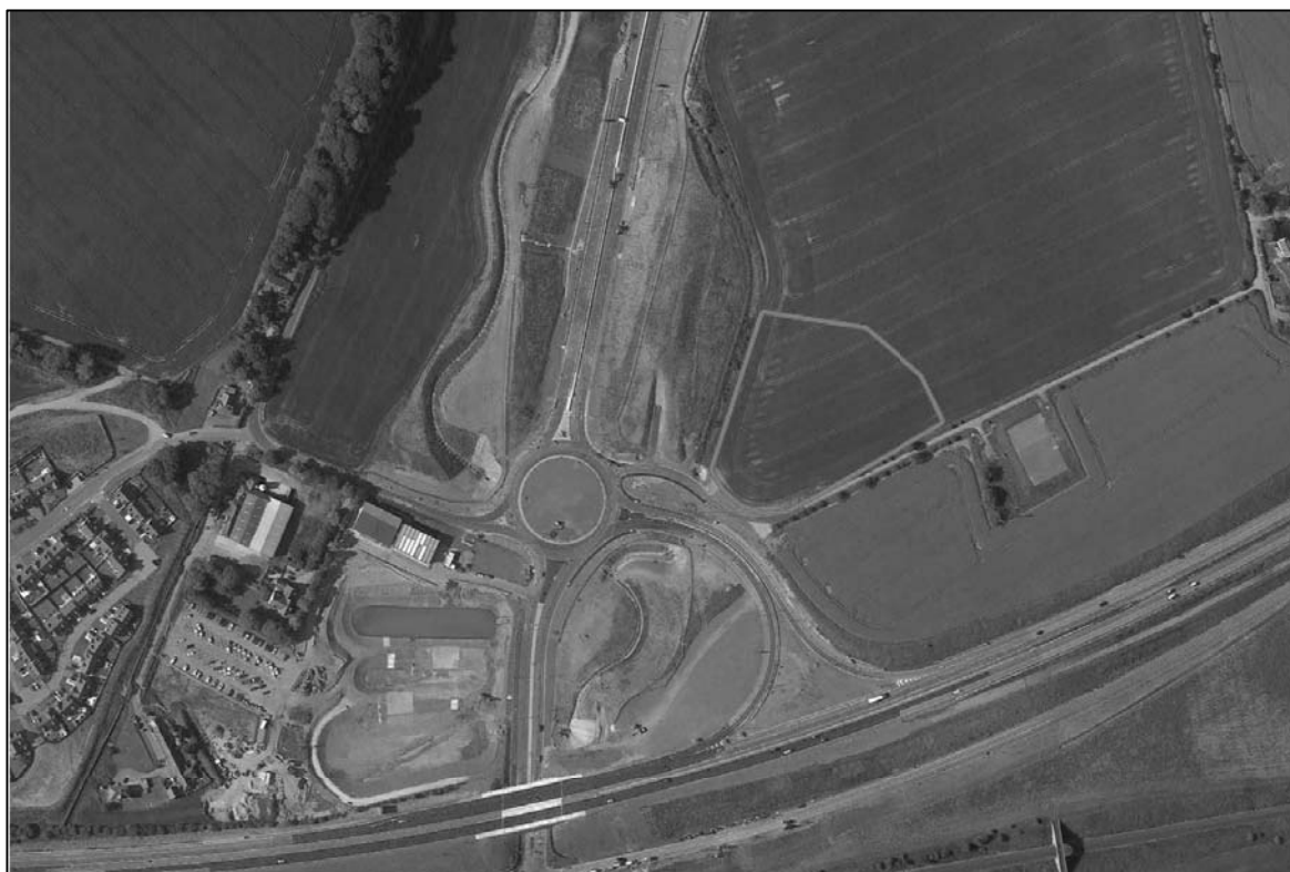
Figure 8 – Aerial Photograph of Site KN119
