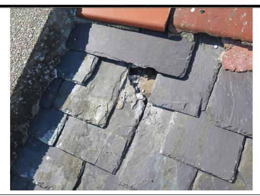
Area of opened up slating to expose condition of fixings / underslating felt.
