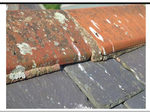
Open mortar pointing below / between fireclay ridge tiles.
