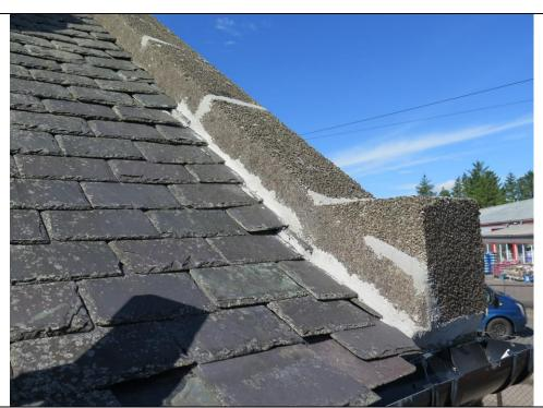
Previous pointing patch repairs to brushed exposed aggregate tabling / coping.
