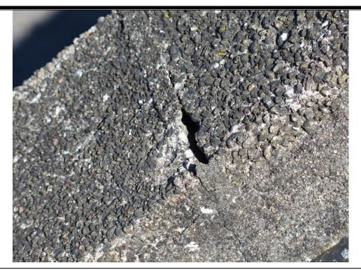
Open pointing in joints in brushed exposed aggregate tabling / coping.
