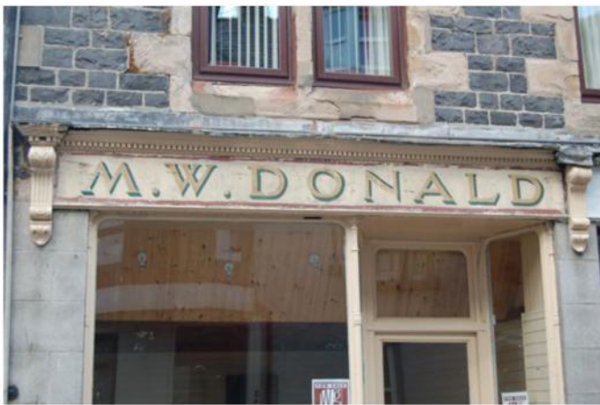
Fig 13 Hand-painted shadow lettering ©Crown Copyright Historic Environment Scotland
