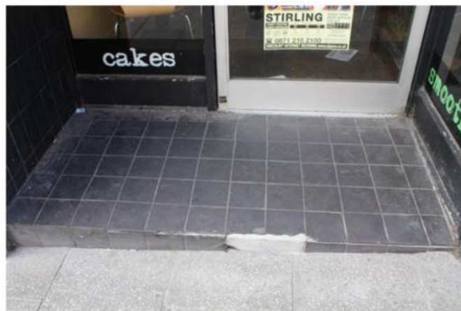
Fig 7: Modern tiles can have a poor appearance and are easily damaged as they lack the robustness of traditional tiles ©Lindsay Lennie
