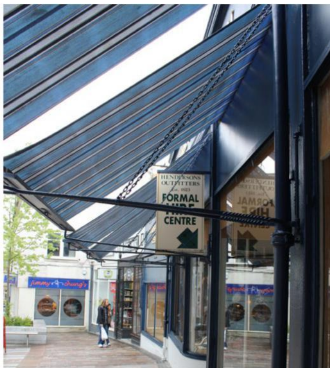
Fig 24 and 25 Traditional awnings can be extended to varying positions depending on the location of the sun ©Lindsay Lennie
