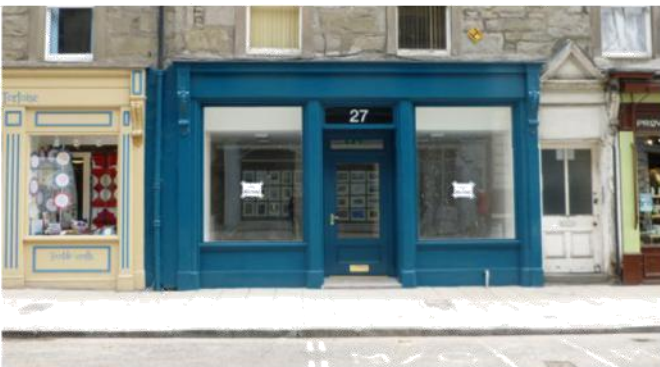
Fig 31 and 32 Stripping back later alterations can reveal the original details as in this example. The Victorian shopfront was uncovered and sympathetic details reinstated. ©Lindsay Lennie
