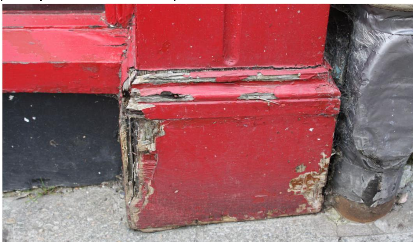
Fig 35 Plinths at the base of pilasters are particularly vulnerable to rot and require regular maintenance, particularly if constructed of timber. ©Lindsay Lennie
