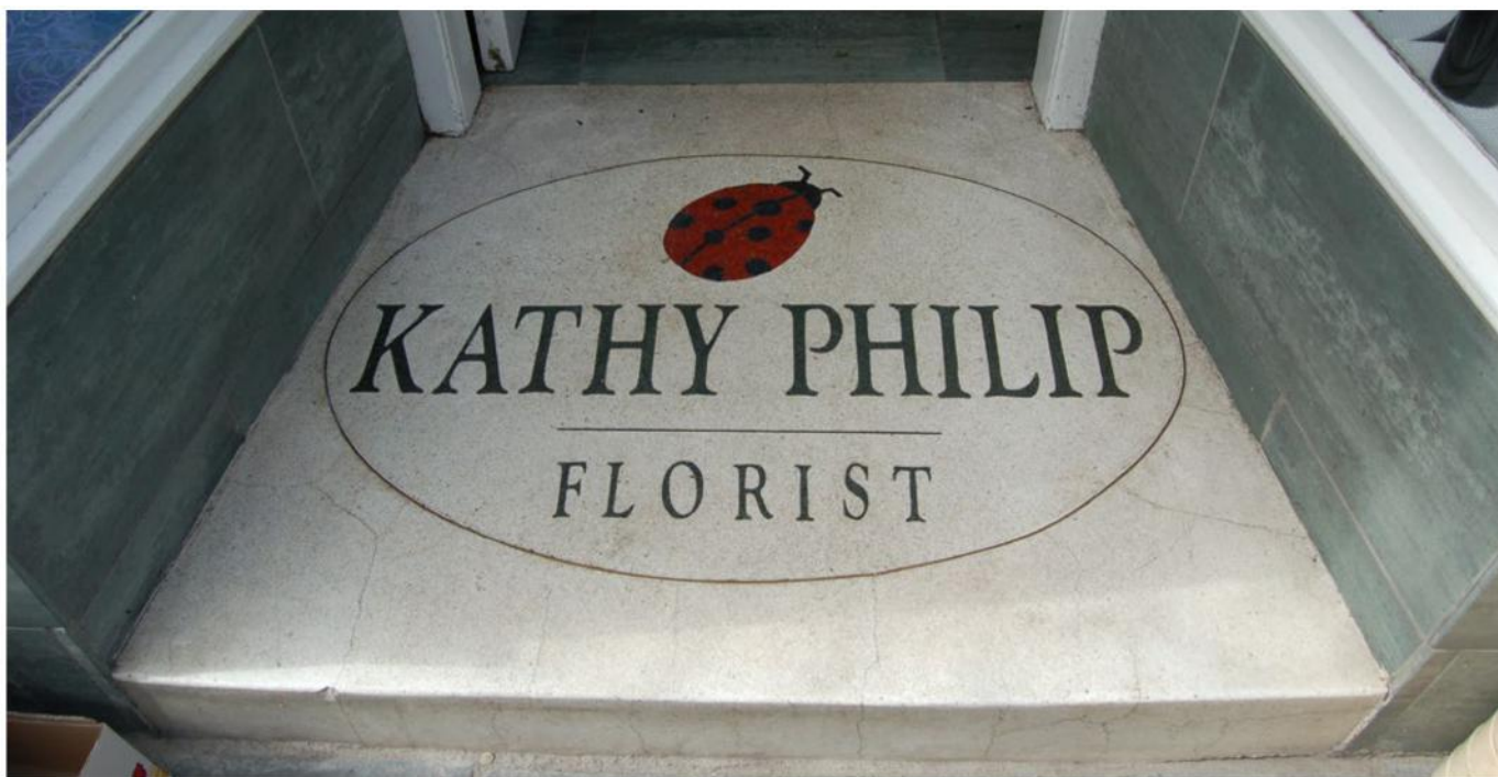
Fig 8: A modern terrazzo floor provides an attractive entrance to a shop ©Crown Copyright Historic Environment Scotland
