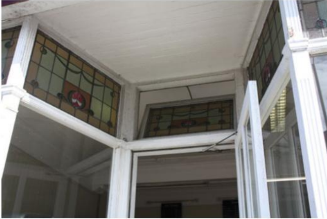
Fig 9 A stained glass clerestory will usually date to around 1900 ©Lindsay Lennie
