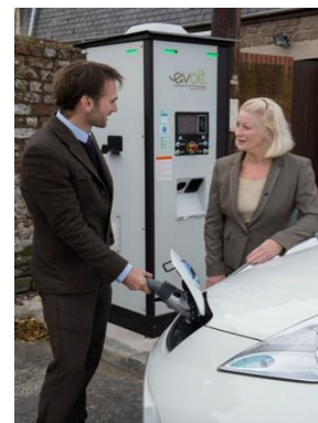
Figure 1.1: Example of a rapid charging point (50kW)
